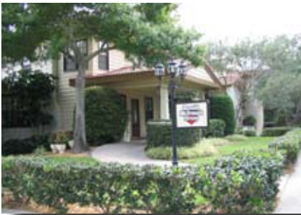
St. Pete West House 18 Bedrooms
